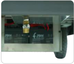
Condensate drain valve
